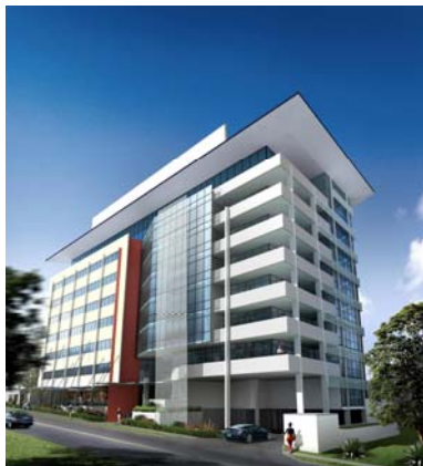
8 level building under construction on 35 Boundary Road, South Brisbane
